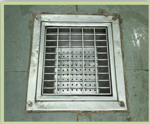
Covered Drains to prevent entry of pests
