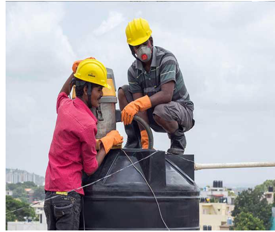
Cleaning of water storage tanks
