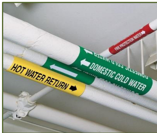
Colour coding of water pipes
