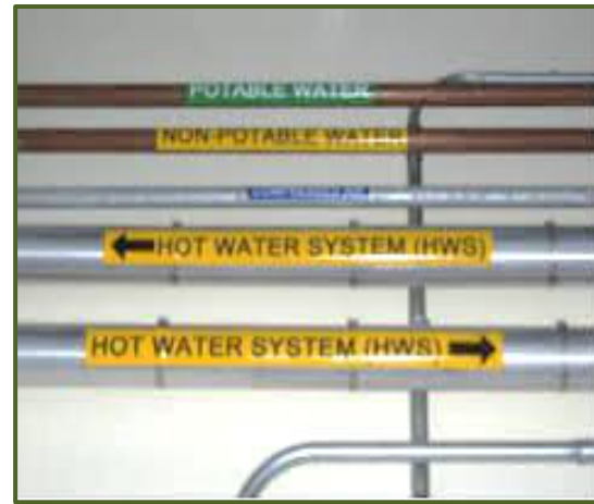
Demarcation of pipelines
